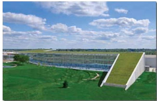
Haworth headquarters in Holland, Mich. is a LEED Gold registered project that includes a green roof completed by Turner Construction Company, a 2010 Green Initiative Champion.
